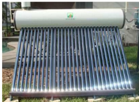
Figure 9.4: Evacuated Tube Collector
