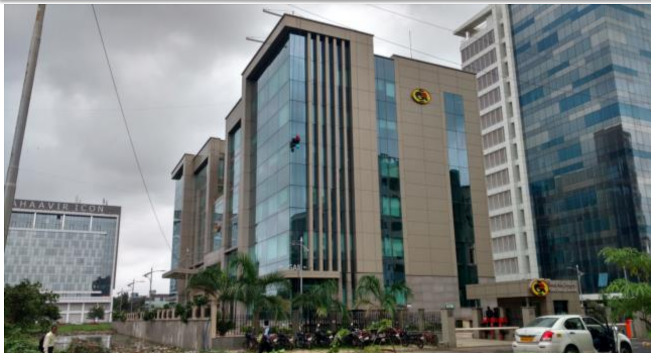
Project GAIL RGMC Office Rating GRIHA 4 Star - Completed
