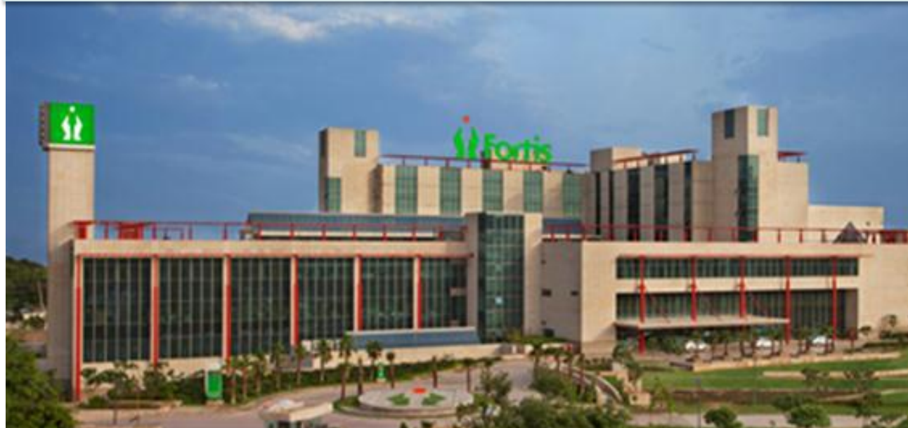
Project Fortis Memorial Research Institute Rating GRIHA 4 Star - Completed
